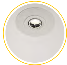
6. Ny innfelt downlight i rehab-ring.
