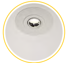
6. Ny innfelt downlight i rehab-ring.
