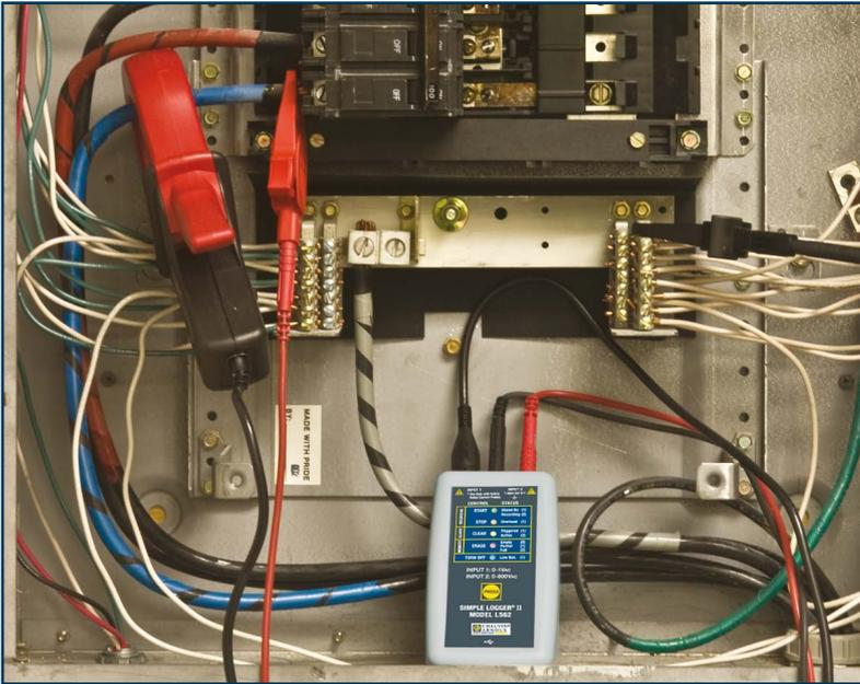
L562 monitoring voltage and current in a load centre.
