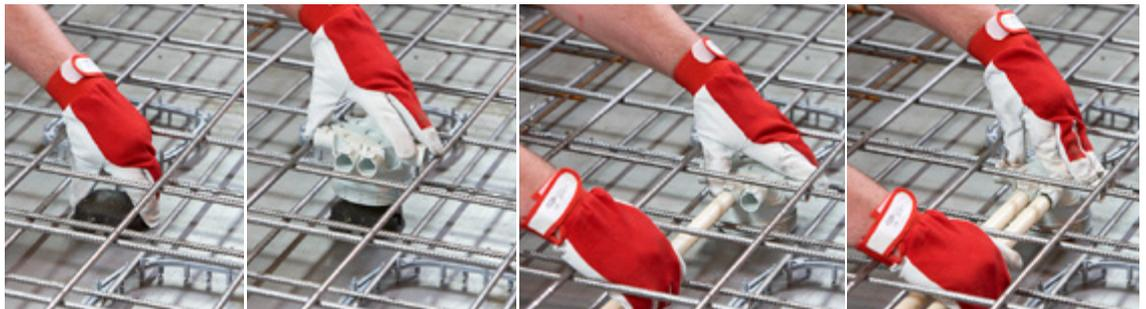
When attaching the boxes to plywood moulds, they can either be nailed or screwed.
