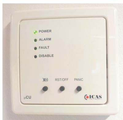
ICAS Micro Control Panel: IMC-Pa, innfelt i vegg
