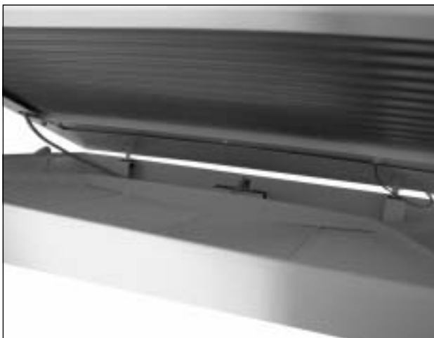
Fig. 41: Install the louvred grille
