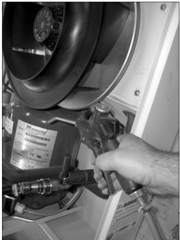
Fig. 83: Clean out the heat exchanger coil and compressor chamber using compressed air (3)
