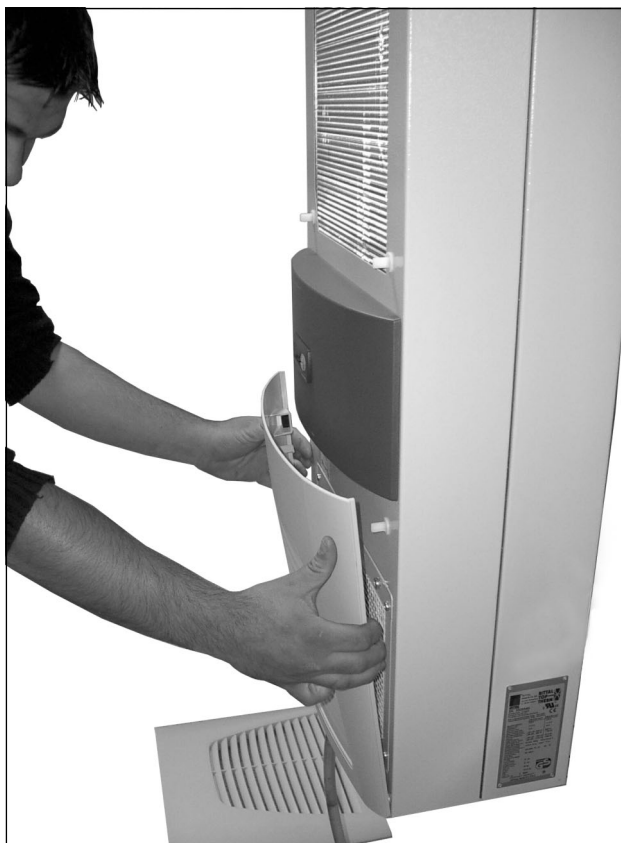
Fig. 43: Remove the lower louvred grille
