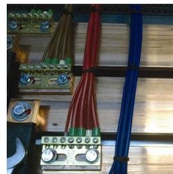
ERICO Connecting, Earthing and Neutral Busbars are used to connect several earthing conductors within a panel and can be used in a variety of different applications including switchgear and control equipment, electrical equipment, for wind and solar power generation and in data centers. This Universal Connecting Bar can be used as a 450A current rating IEC for power distribution.
