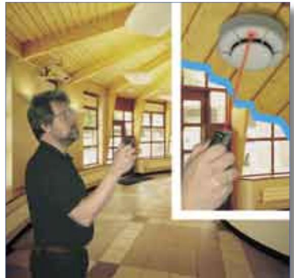
Routine testing has traditionally involved physical access to the installed unit, a time-consuming procedure often requiring the use of step ladders or long poles. The ECO1000 is tested from ground level using a laser based remote alarm test unit. The commissioning or service engineer directs the modulated laser beam at the detector's LED; the unit responds to the commands and latches into alarm. What could be simpler?
