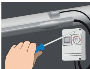
7. Attach and cover the sensor and the tip on top of the pipe with aluminum tape. Extend cold tails/leads and keep connections dry. Mount connection box on the pipe or close to it and install the thermostat on the pipe or near it (depends on thermostat).
