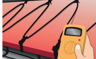
6. Install the cable(s) on the roof, in gutters and downpipes. Check once again and compare the insulation resistance.
