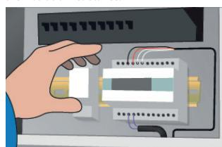
9. Install thermostat/controller and connect cables to the connection boxes and to the switchboard.
